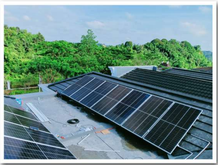
@ Samarinda - 10 kW On Grid 3 phase
